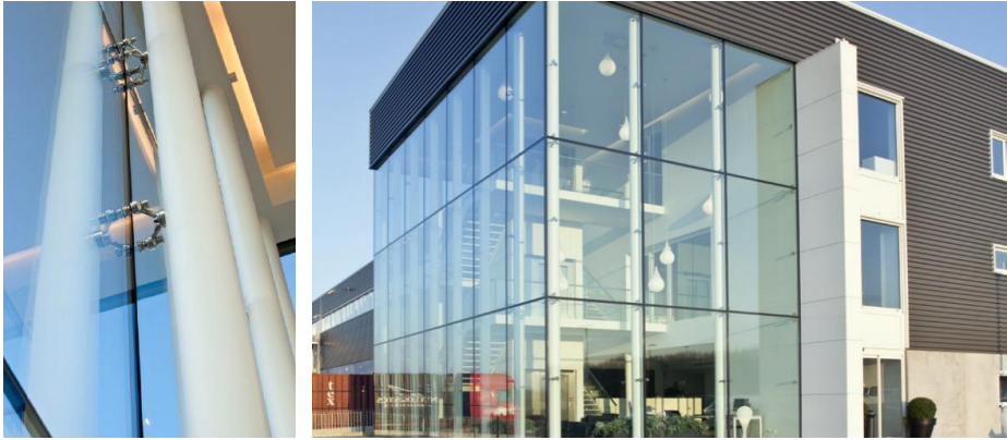
FIGURE 2.15: DOW CORNING EUROPEAN DISTRIBUTION CENTER, EURIDICE WAREHOUSE, FELUY, BELGIUM, ADHESIVE PRODUCER: DOW CORNING (PHOTOS COURTESY OF DOW CORNING).
