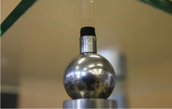
FIGURE 5.2: DISCRETE POINT-FIXINGS WITH A DIAMETER OF 10 MM.
