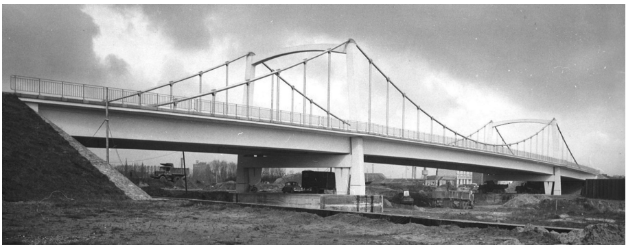
Fig. 1. Self-anchored prestressed suspension bridge with a central span of 100 m at Merelbeke (near Ghent).
