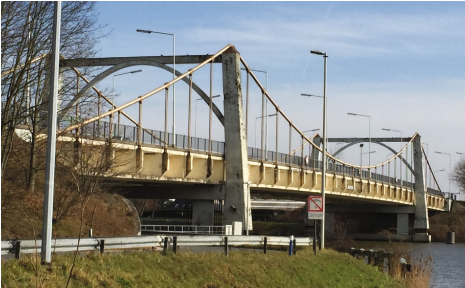
Fig. 9. Bridge at Mariakerke (W16).
