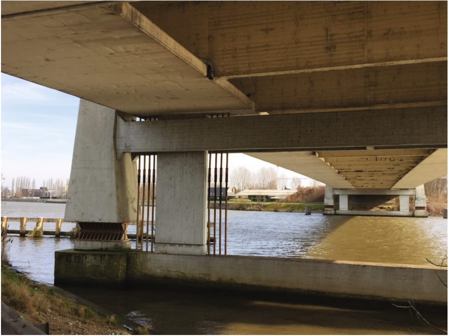
Fig. 10. Lower part of one of the piers of bridge W16.
