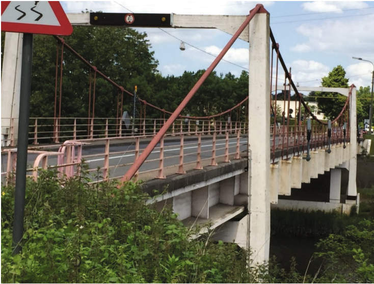
Fig. 7. First self-anchored suspension bridge designed by Vandepitte (W13).
