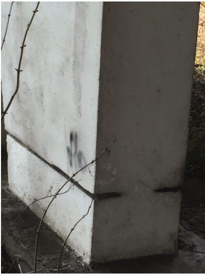
Fig. 4. Freyssinet hinge at lower part of V-shaped bearing wall.
