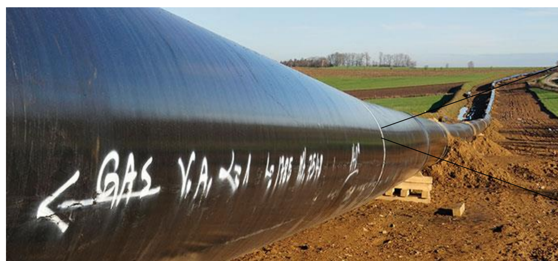
A welded oil pipeline
