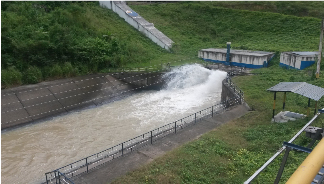
Figure 3.2 Picture taken at the tailrace of the Poza Honda hydropower dam.
