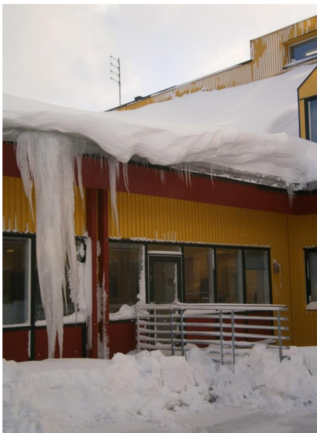
Photos from the SANA hospital in Nuuk, taken in the February (left) and in May. The pictures show how a heavy layer of ice is built up under the snow during the winter. This layer can obtain a considerable thickness with very large icicles. The picture from May shows what can happen by the thaw, when such an icicle and block of ice break loose and fall on a staircase / ramp. Besides being a danger to the surroundings the massive ice means a risk of damage to the roof and deformation of the overhang.
