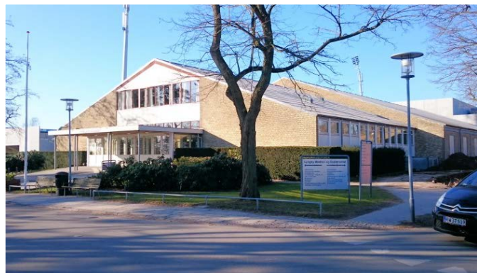
Picture 6: Lyngby Idrætsby main entrance
