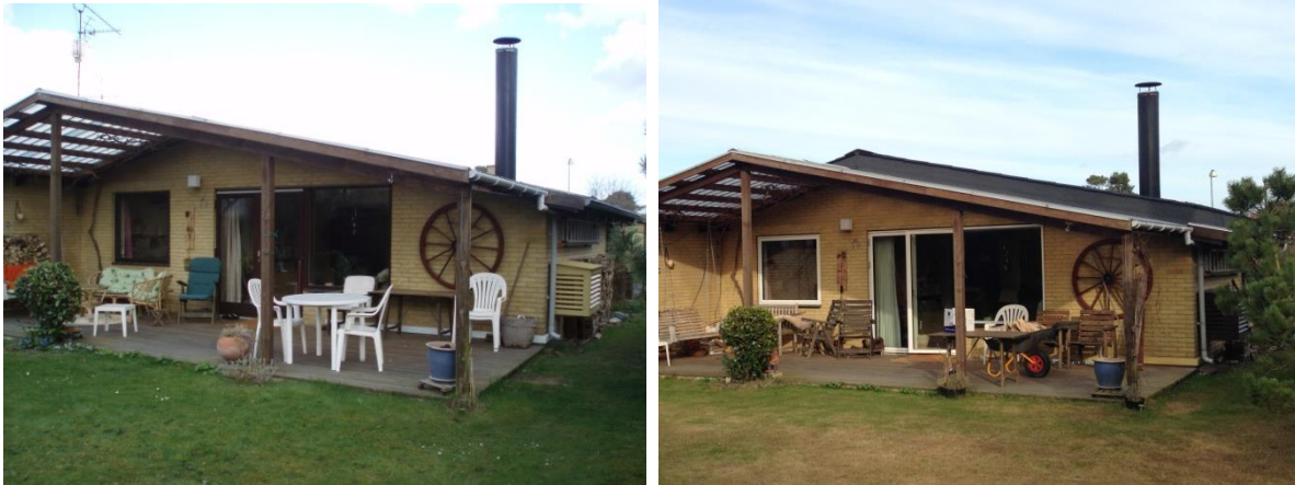
Fig. 9. House A before and after the renovation. Visible changes are the new windows and roof.
