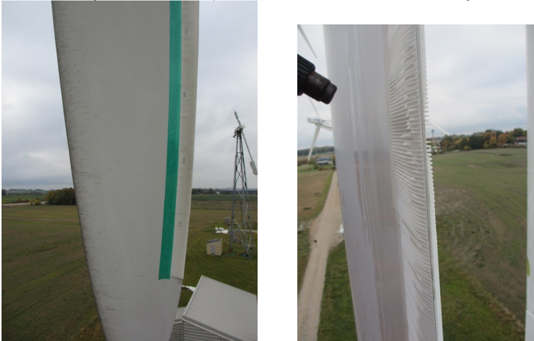
Figure 8 - Finlets installation set-up
