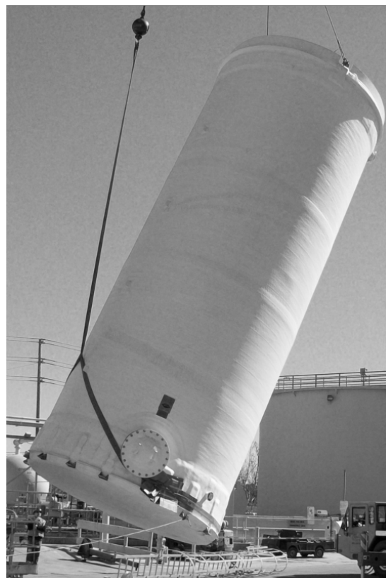
Figure 13: Example of a FRP tank made of Derakane vinyl ester [74]. Courtesy of Ashland Inc. and Owens Corning
