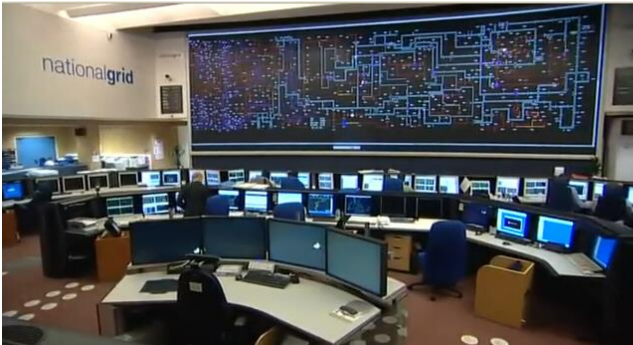
Figure 4—1 Example of TSO control room (National grid, UK)
