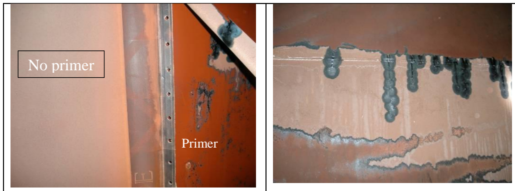
Figure 8: Duct before booster fan (left) and duct before silencer (right).
