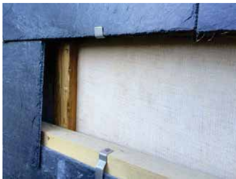
Figure 3: The MgO-board is placed facing the air gap, which is behind the siding boards made of natural slates.
