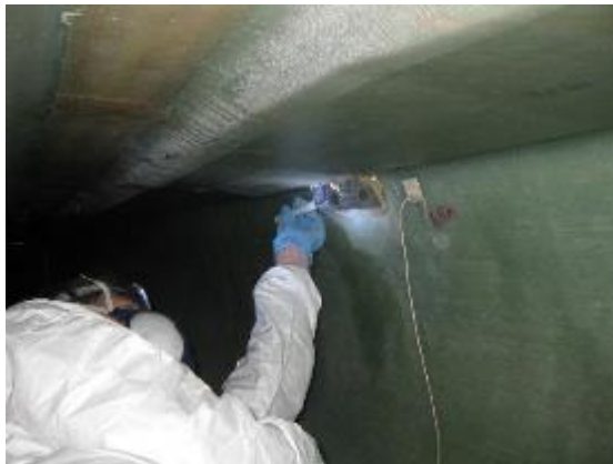
Figure 122 – Installation of X-Stiffener in 15m section
