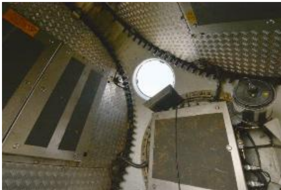
Figure 34. Entrance to the hub.
