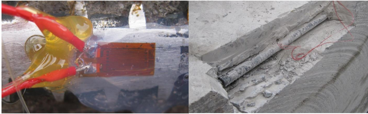
Figure 5, (left) photo of a strain gauge mounted on a reinforcement bars – (right) photo of a cut reinforcement bar
