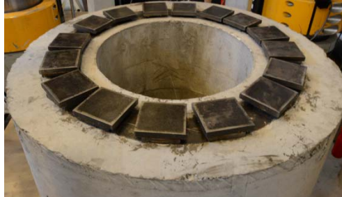
Figure 11: Sandwiches of steel plates with grease in between placed on top of the concrete base for support of the sleeve.
