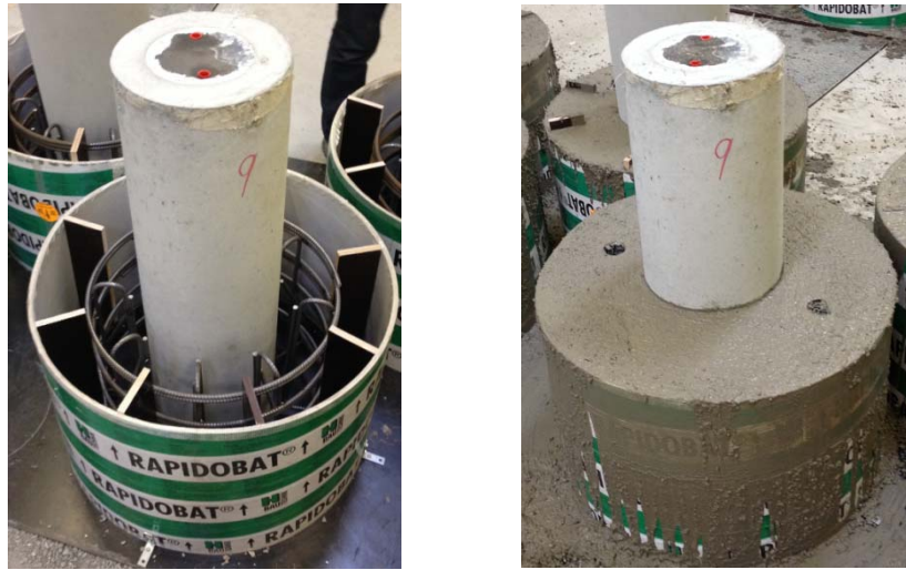
Figure 5: Piston, stirrups and crack inducers placed within sleeve formwork (left) and buffer system after casting of sleeve (right)
