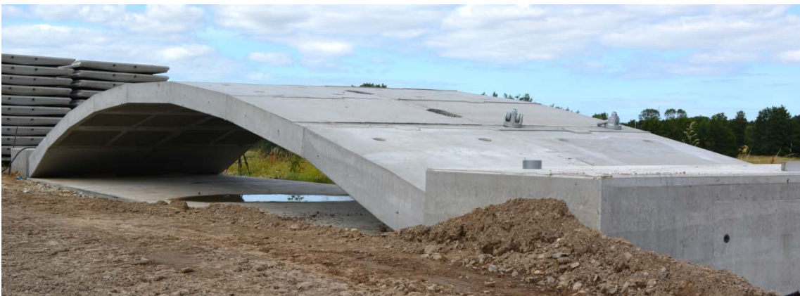
Figure 2: Two adjacent PC-Arches after assembly and lifting.
