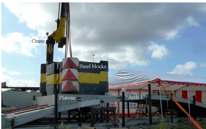
Figure 11: Test 1. Six steel blocks, each weighing 10 tonnes, were set on the plateaus on “arch 1” (near side in photograph) and “arch 2”.
