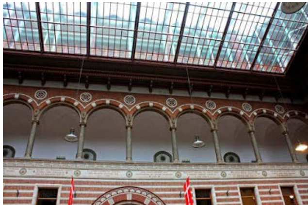
Figure 16. Photo Case A Borrowed from the official website of the municipality
