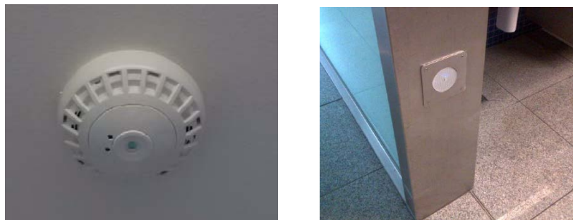
Figure 8. Sensors detect people entering the room Left photo: Thermal sensor above door. Right photo: Light sensor in door opening.
