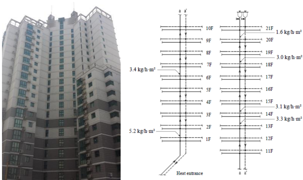
Figure 3. Building #3's appearance and the mass flow along one of the vertical riser supplies(Zhang et al. 2016)
