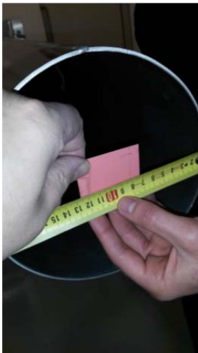
Figure 70 Checking the centre
