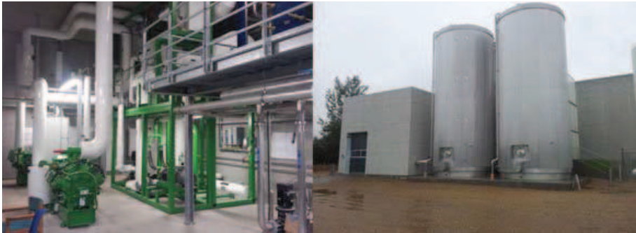
Figure 1.1: HACHP at Arla's powder milk factory Arinco in Videbæk, Denmark.
