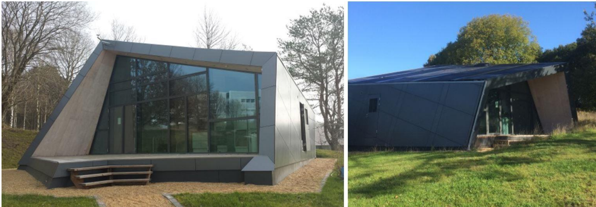
Figure 1. Exterior views of the house, seen from North-West (left) and South-West (right)
