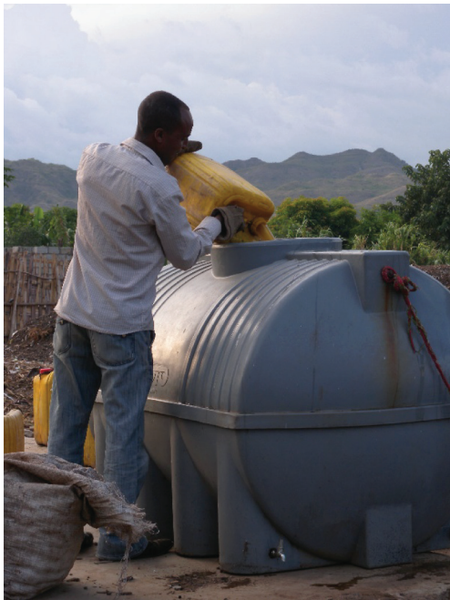
Figure 2 Urine collection tank in Arba Minch, Ethiopia (picture: Elke Müllegger, EcosSan Club, Austria).
