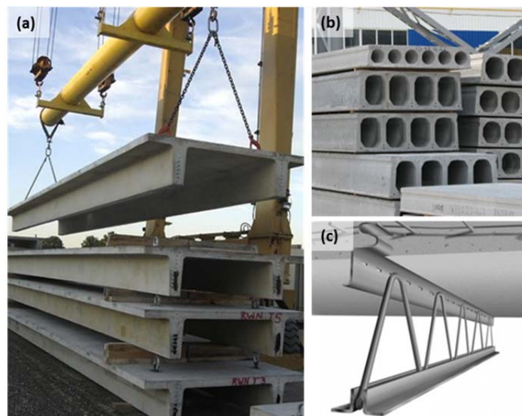
Figure 8.1 Commonly used prefabricated structural panels: (a) double-T panel ( www.stubbes.org ); (b) hollow core panel ( www.oberbeton.com.ua ) and (c) Hambro panel (Hambro 2009)
