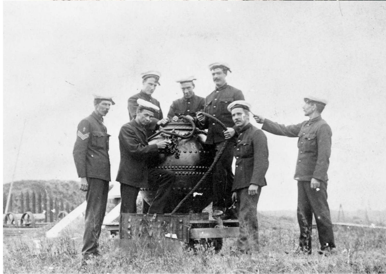
Above: 1880 Plan of Lytton Battery Reserve stamped by F.D.G. Stanley, architect. Fort Lytton Collection Opposite: Nineteen members of Queensland Defence Force Artillery standing on top of Armstrong Disappearing Gun Shield at Fort Lytton Gun Pit One circa 1890's. Fort Lytton (Fred Parker) Collection Submarine Miners pose with a 100 pounder mine circa 1900. Fort Lytton Collection
