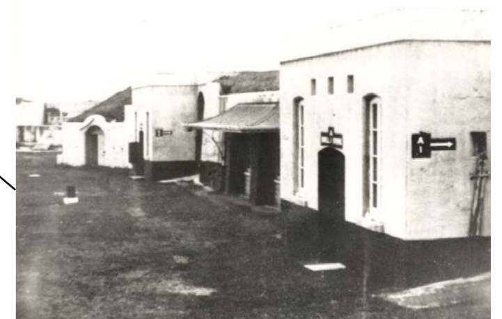
1936 view of parade ground with Casemate One in foreground, the magazine stores and Casemate Two. Fort Lytton Collection
