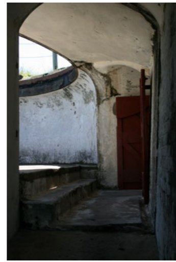
Entrance into gunpit #1, originally built in the 1880s. UQ, 2016
