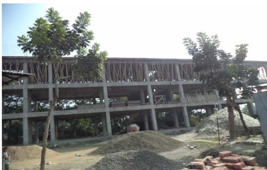
Figure 7.5. Cyclone shelter under construction in Kacha.
