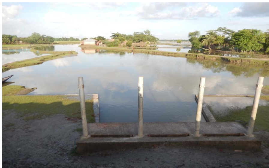
Figure 5.3. Sluice gate and canal to control and store water
