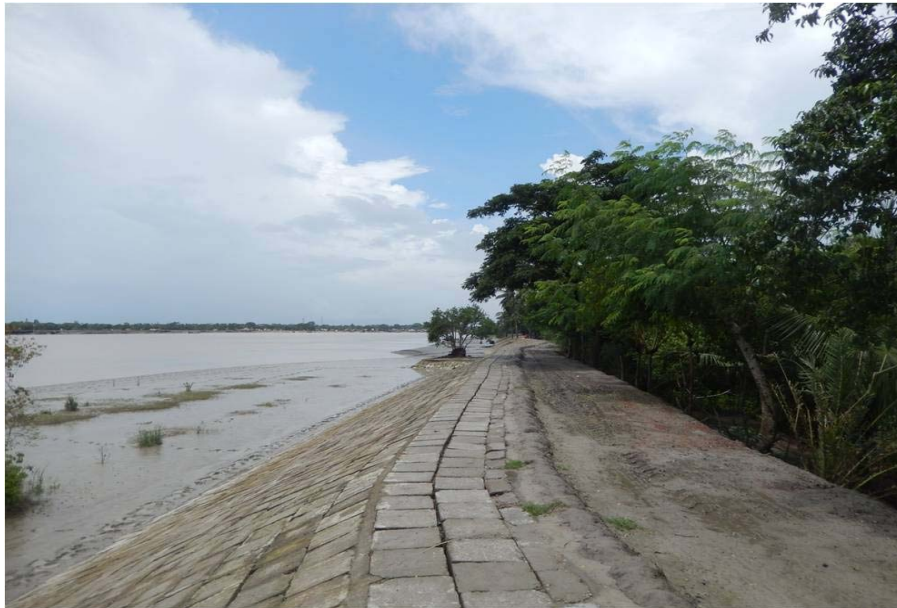
Figure 5.2 Embankment to protect farming land and villages
