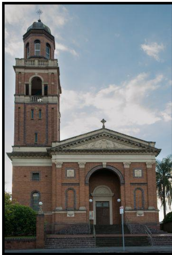
Figure 4.3. Holy Spirit Catholic Church, New Farm (1929-30)
