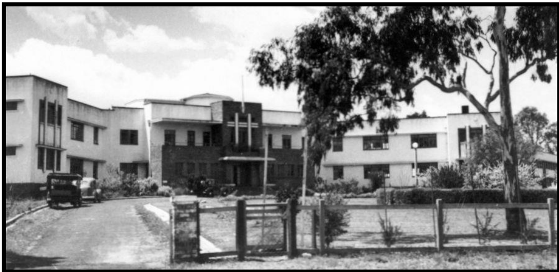
Figure 5.2. Kingaroy General Hospital (1938-39, altered)
