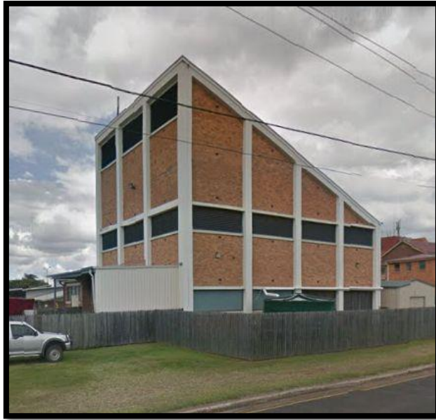
Figure 6.8. Boiler House, Maryborough Base Hospital (1956, altered) Now the Services Building
