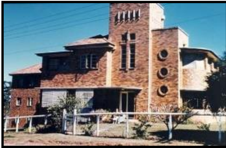
Figure 5.5. Nurses' Quarters, Nambour Hospital (1941-42, demolished)
