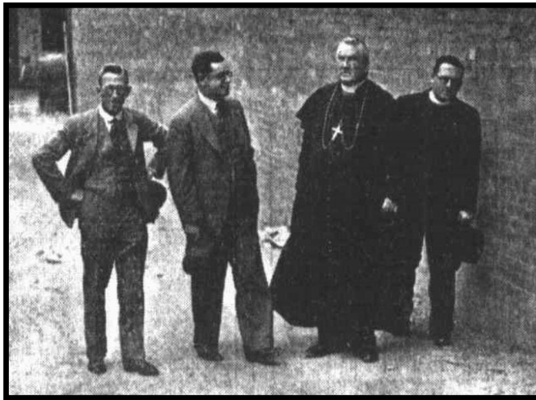
Figure 4.1. Donoghue (second from left) and Duhig in 1937 Inspecting work on Ozanam House
