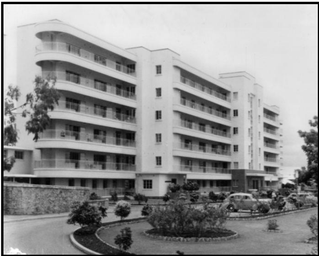
Figure 5.6. Townsville General Hospital (1945-51, now a residential complex)
