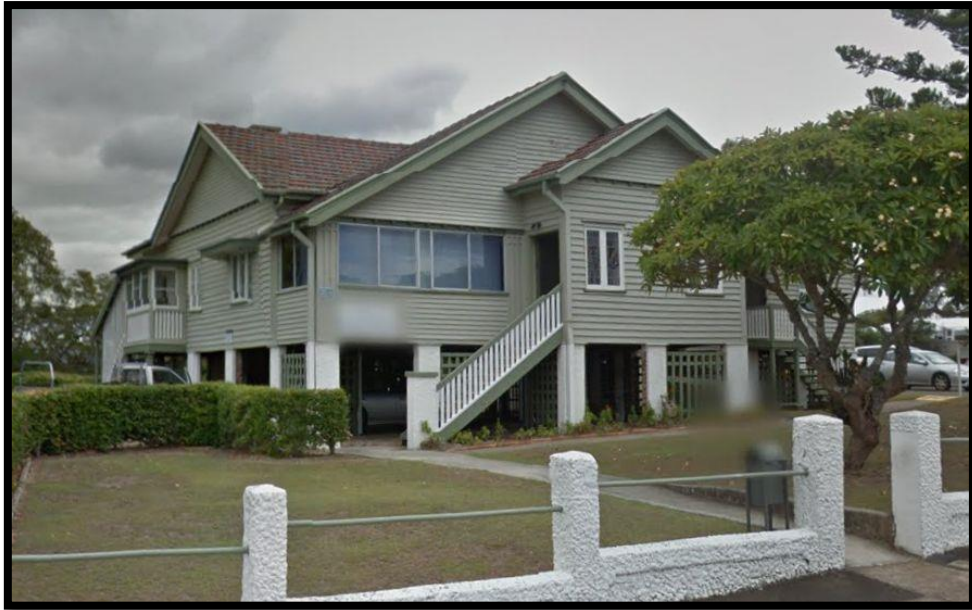
Figure 4.14. Presbytery for St Joseph's Parish, North Ipswich (1934)
