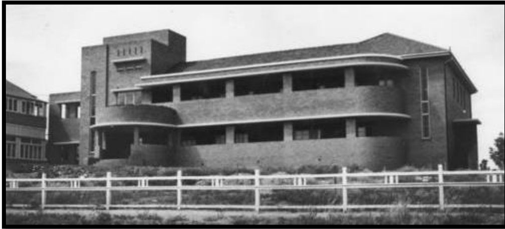
Figure 5.3. Warwick Maternity Hospital (1938-39, demolished)
