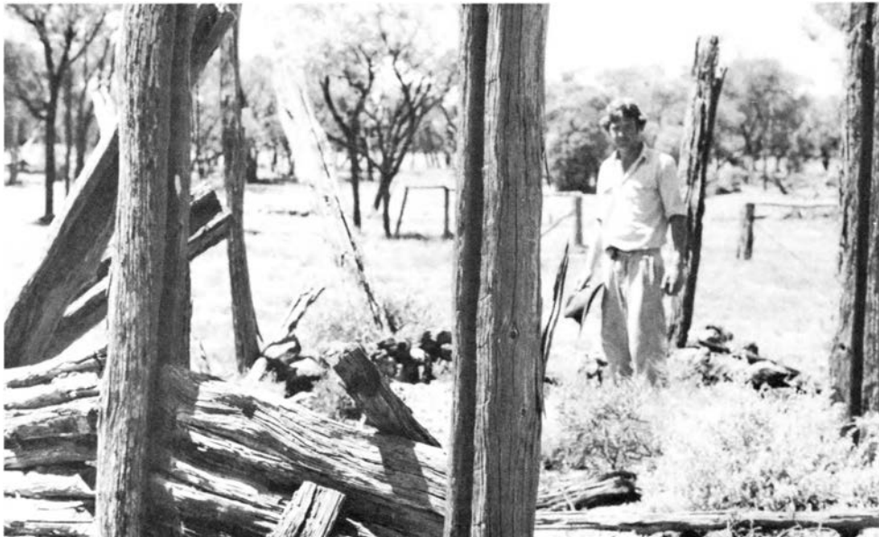
Ruins of one of the old huts on Boondoon. The author's youngest son, Richard, is standing at rear, beside an old stone fireplace. Note the deep slots in the gidyea posts, into which the tapered ends of the horizontally laid slabs fitted.
