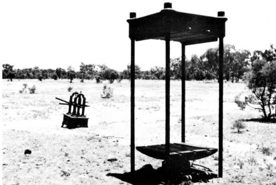
Remains from Sidney Yeates' time (1881-1894) on Boondoon in the woolshed area. Upper photo: stone fire places which probably formed parts of the shearers' quarters and bake-house. Lower: huge iron dumper for compressing wool bales, with nearby machine which may have been the dumper's winding gear.
