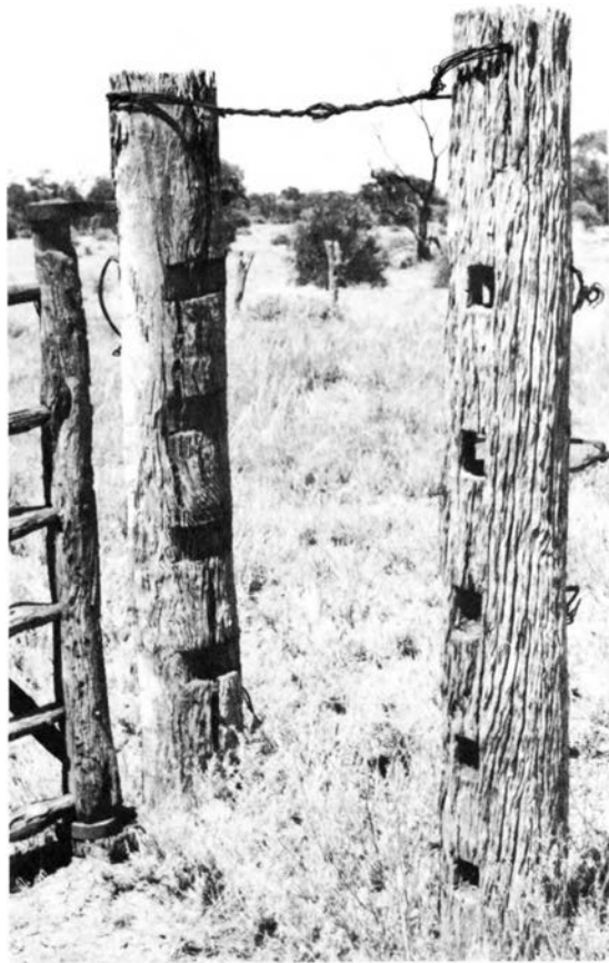
Many post and rail cattle yards, made from the local gidyea, still exist on Boondoon after more than a century. Upper picture: one set of yards still in use to-day. Lower: close-up of gateway construction.
