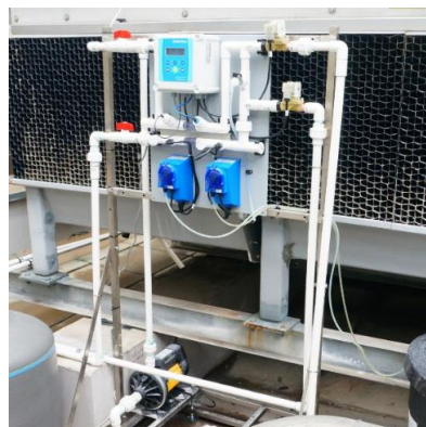
FIGURE 6-3 THE CHEMICAL TREATMENT FOR PLANT ROOM FIGURE 6-4 BYPASS CHEMICAL SHOT FEEDER TO PREVENT CORROSION IN CHILLED WATER
