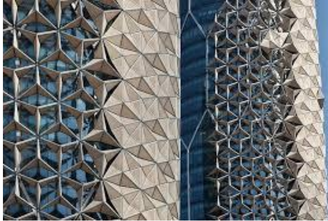
Figure 4 - Actuated, folding facade of AL Bahar Towers (Source - http://www.archdaily.com/270592/al-bahar-towers-responsive-facade-aedas )
