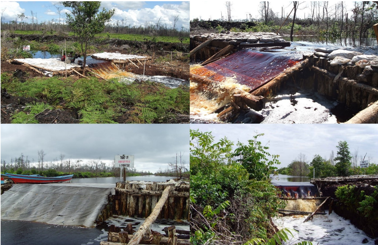
Figure 3.8 Dams with spillway system constructed in the EMRP, Central Kalimantan
