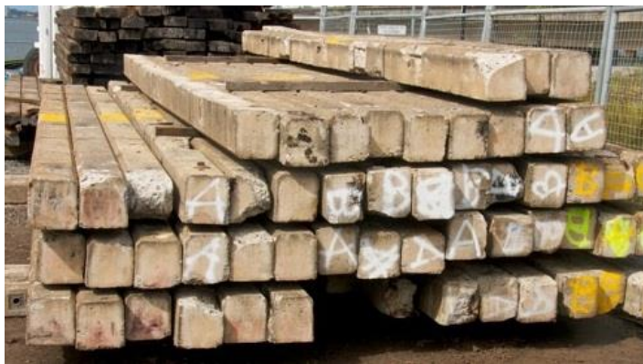
Figure 1 Sample piles after demolition showing no exterior evidence of internal corrosion.
