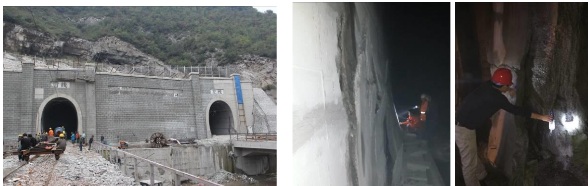
Figure 1 Profile of the tunnel, extruded 2nd lining and surrounding rock water collection
