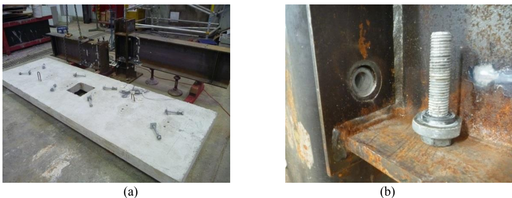
Figure 8 (a) Specimen CJ4 dismantled by removing the bolts and (b) unbolting of blind bolt.
