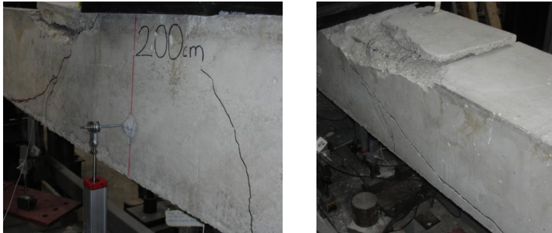
a. steeper cracks close to east support b. inclined cracks close to the west support Figure 6 Inclined shear cracks
