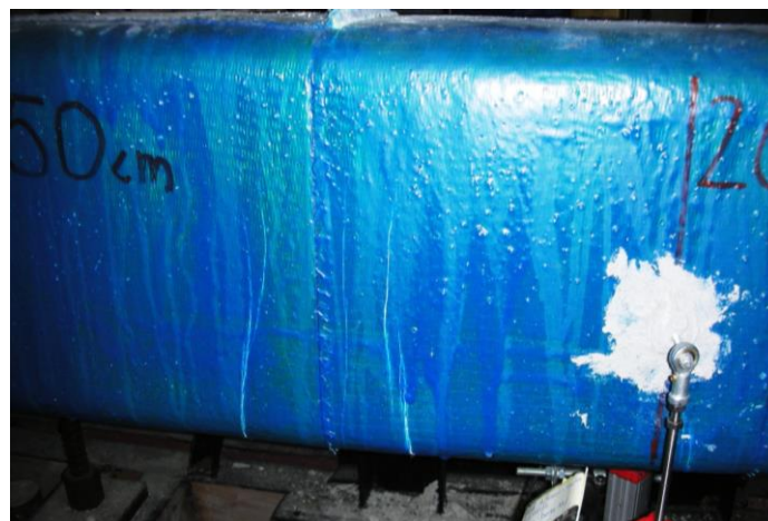
Figure 9 Cracks of ImpA1 after the first impact
