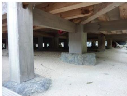
Photo 2 Post erected on a foundation stone
