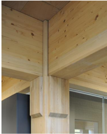
Figure 3 a) Joint between the column and the beams b) Installation of a load cell (tendon anchorage point)
