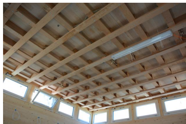
Figure 2 a) Beech plates for the timber-concrete composite floor b) Bi-axial timber floor in beech wood
