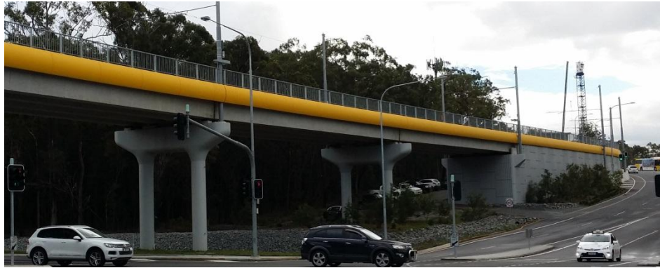
Figure 1 Picture of typical highway bridge
