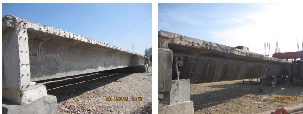
(a) Girder before reinforcement (b) Girder after reinforcement
