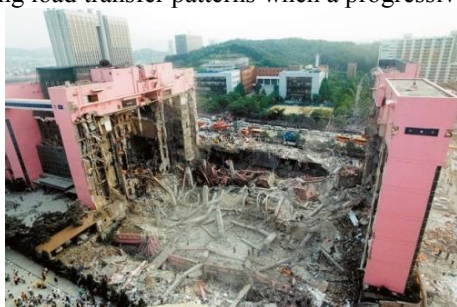
(a) Sampoong Department Store collapse (Park 2012)
