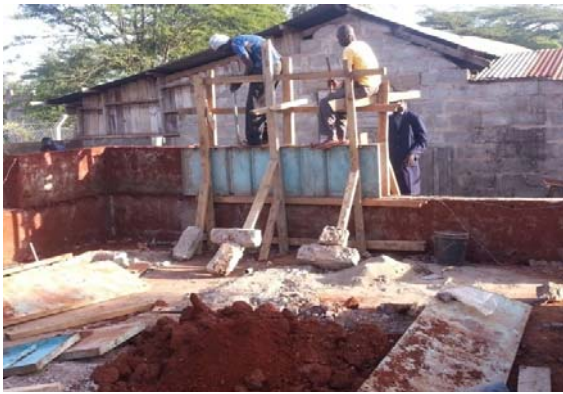
(a) Ramming process of earth wall
