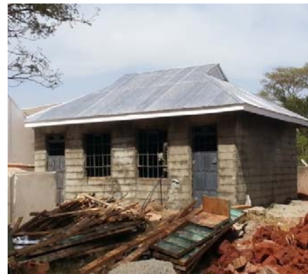
(b) Model single storey rammed earth building
