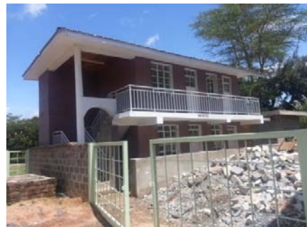
(b) Completed structure under use as office block
