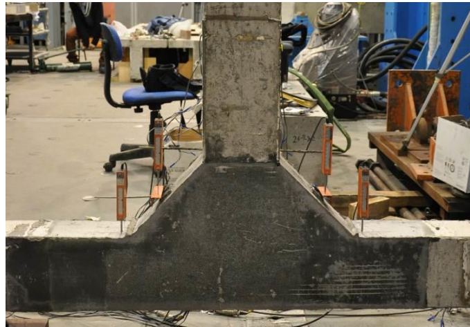
Figure 2 Exterior beam-column joint strengthened by ferrocement jackets with chamfers
