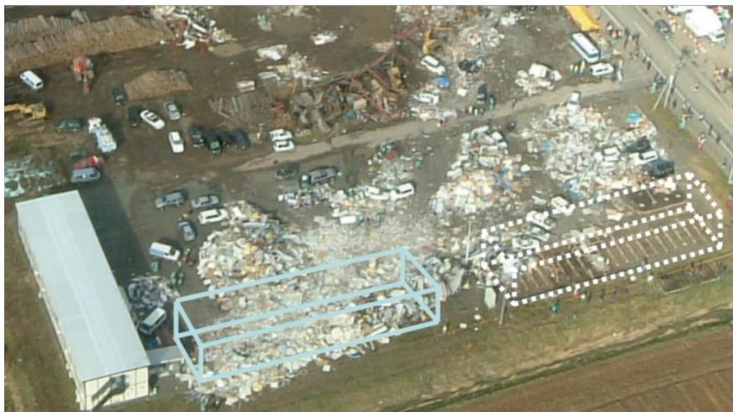
Figure 6 Damage to construction work offices due to a tornado in Saroma-cho, Hokkaido, Japan, on November 6, 2006 (Tamura et al. , 2007)
