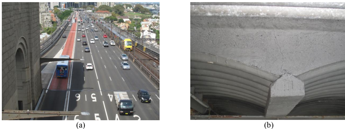
Figure 1. Illustration of (a) the bus lane on the Sydney Harbour Bridge, (b) one of the concrete jack arches underneath the bus lane.
