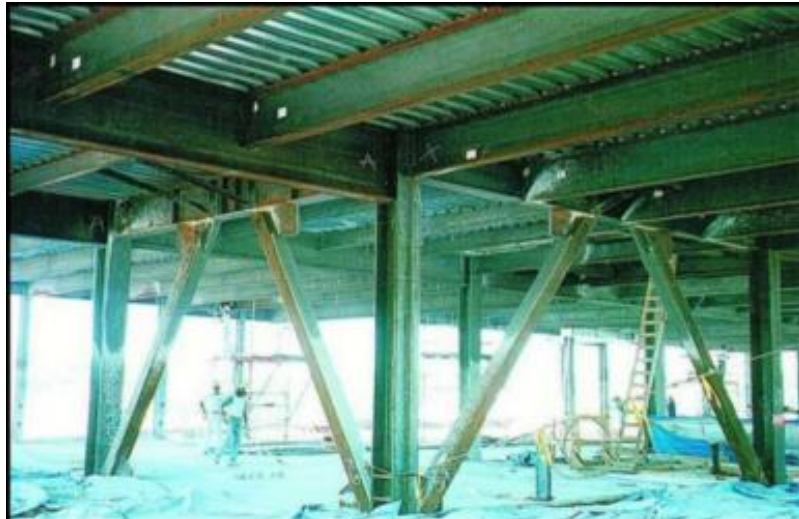
Figure 1.2 Building with EBFs (Ogren engineering Web page)
