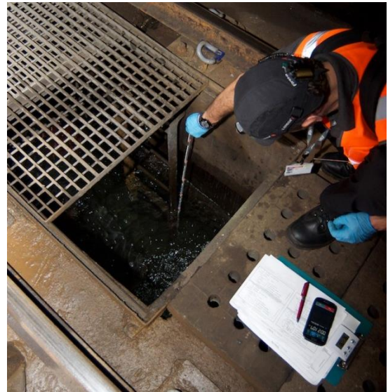
Figure 5: Measuring the sump water level
