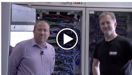
Movie 5.1 Demonstration of a server room.
