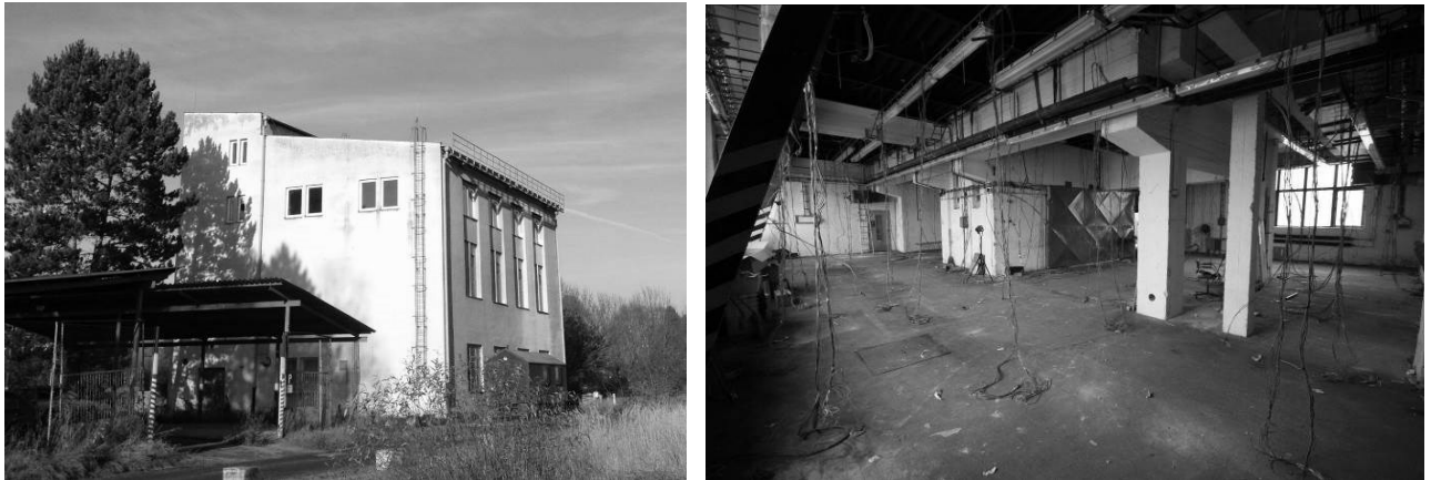
Figure 1: Left – Southwest corner of test building, and Right – fire compartment
