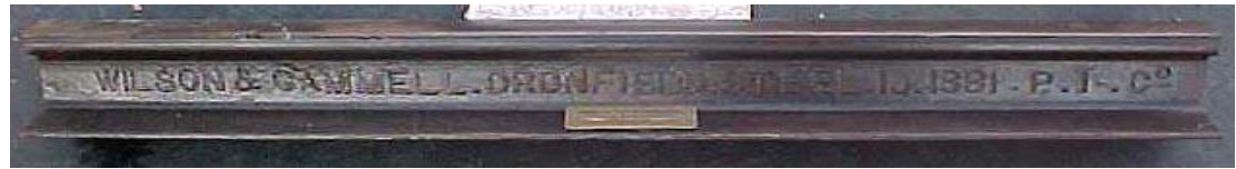
Wilson Cammell & Co, Dronfield - ~1860s
