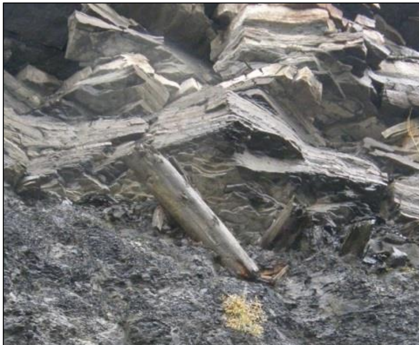
Figure 33: Wooden pit prop in situ within the Muirkirk Nine Foot coal workings. The wooden props were used to hold up the roof of the workings as the coal was extracted. The prop, sitting above packed mine waste in the photo, has since collapsed due to the overlying weight of rock above.
