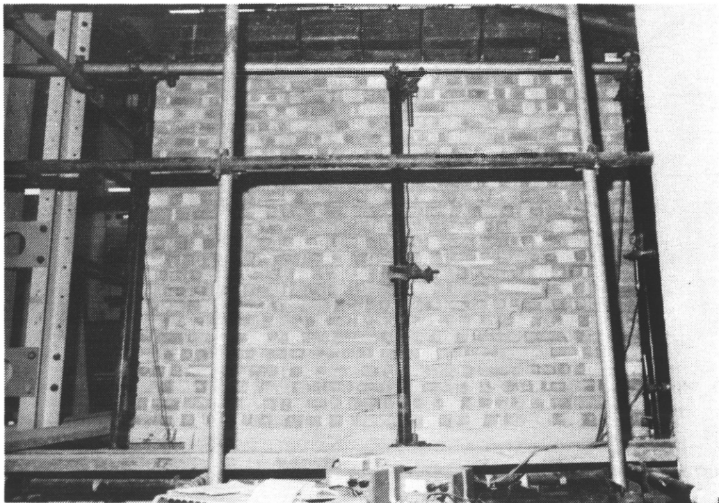
Figure 8.64 Diagonal cracking at lower courses of wall during settlement (Test W5).
